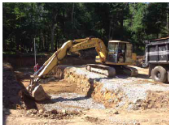
Peter McEachern Excavating for the Farm's Manure Storage Shed
